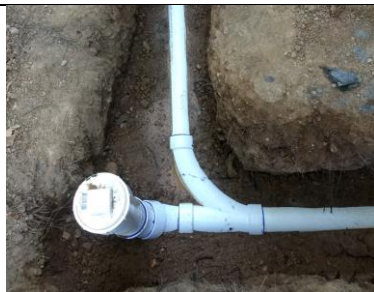
Gravity Main and Lateral Connection
