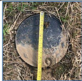
Service Box/Valve Pit
