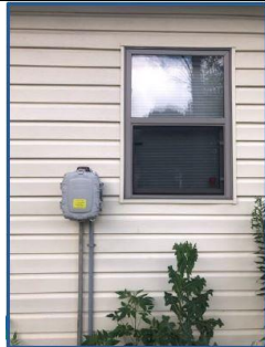
Installed Control Panel
